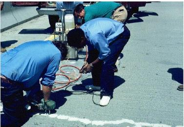
Figure 31. Epoxy Injection Procedure (VirginiaDOT 2009)
