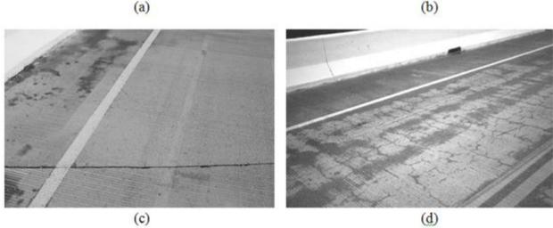
Figure 28. Types of bridge deck cracking: (a) transverse, (b) longitudinal, (c) diagonal, (d) map (TRB 2004)
