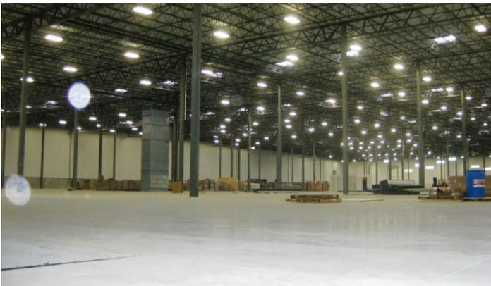
Lorne Seifert chose to use a 4000 psi 467 concrete mix for the slab and facilitated its placement with a laser screed. Typical slab placement would begin at midnight and the average pour size was 1000 yards. The wall slabs would often overlap slab placements, which resulted in DVC often supplying both concrete subs simultaneously.
